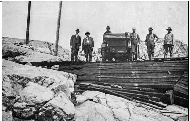
Unidentified "autoists" crossing on top of the Donner Summit snowsheds. When the snow covered the barn doors that allowed vehicles to cross the tracks by going through the sheds, or later the snow covered the underpass, this was the only alternative to waiting for snow melt.
