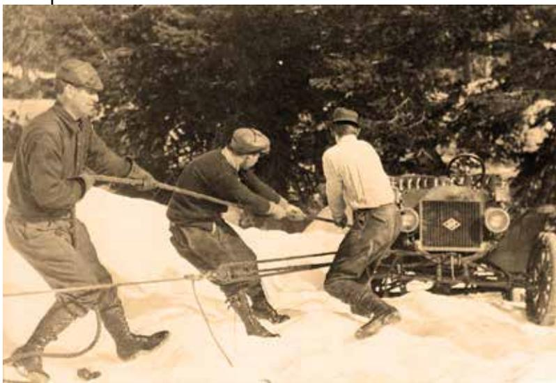
Note the 150' of 1" rope wrapped around the tires to give the car better traction.
