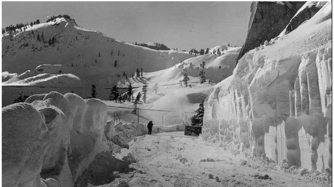
and rocks that have slid down and been buried in the drifts. When the augurs on a rotary hit a rock, a small shearing pin breaks to save the heavier machinery and the crew must get out into the gale, take off their gloves and put in a new pin with their blue hands. Three times in an hour... A brand new rotary is almost ready to go from the State's garage in Sacramento. "All it needs now is a coat of paint," he is told.
