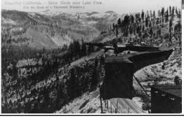
snowsheds circa1910. These were telescoping snowsheds. Parts were on tracks that enabled the sheds to be opened in winter and so stop fires. The sun baked wood was quick to catch fire from snokstack sparks and then the sheds acted like chimneys. Fires blazed into conflagurations and miles of sheds could be destroyed in one fire. Fire trains were always at the ready and track walkers conintually inspected for fires.
