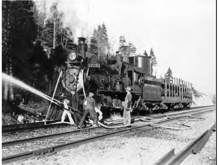
Fire train in action
