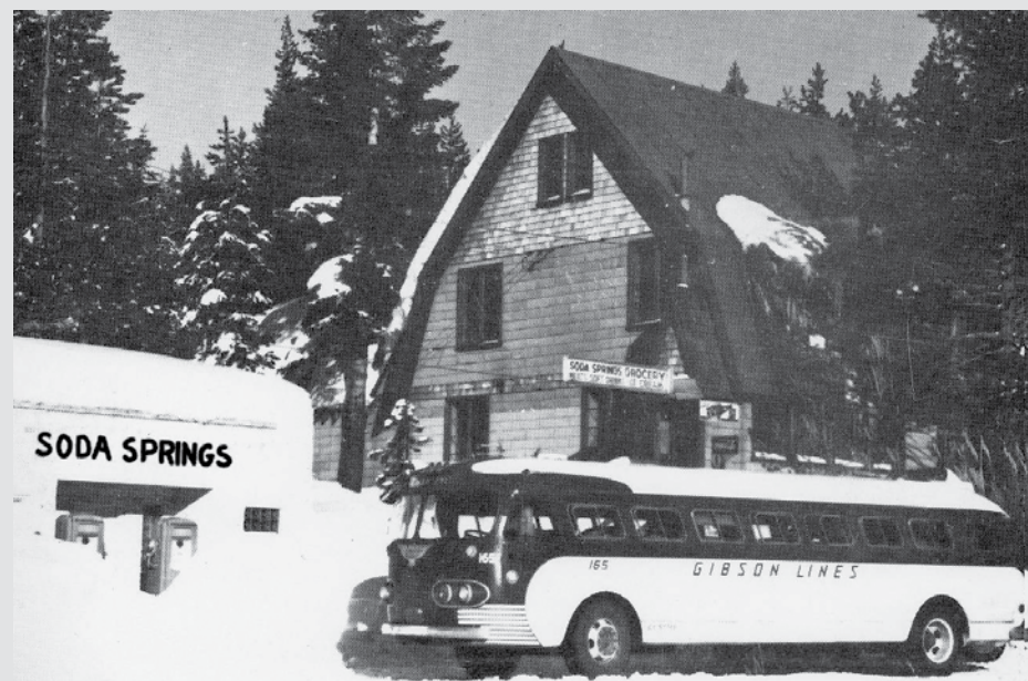
Soda Springs Grocery, the large building behind the bus.
